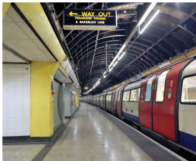
The Jubilee line terminus at Charing Cross (now closed). Photo Nick Catford
